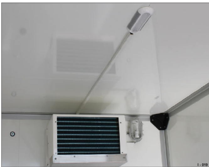
Fig. 28 Luz LED de 12 V com interruptor
